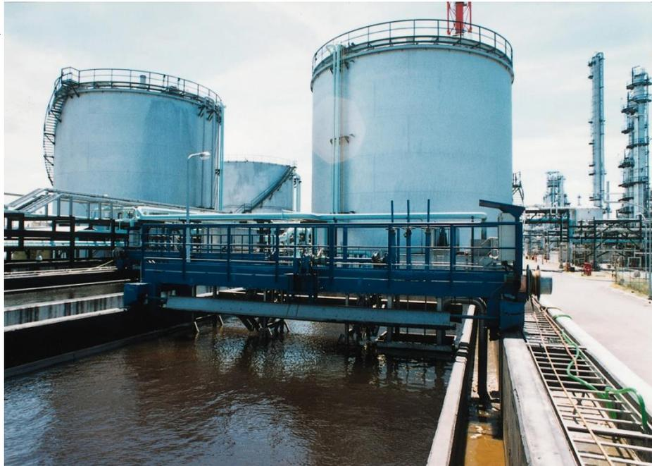
Taiwan Prosperity Chemical Corporation treats its phenol production effluents in an in-plant biological wastewater treatment system. To provide maximum operating flexibility, the wastewater treatment system is built in two lines which can be operated either in parallel or in series.
